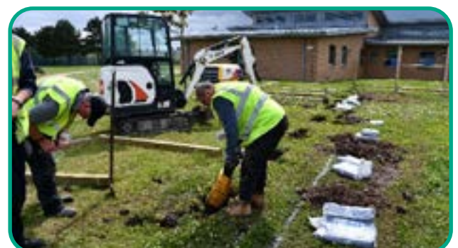
Women's Service Construction
